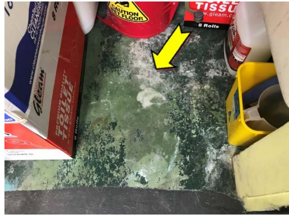
Photo 4. Interior, female toilets, store cupboard, floor – suspected lead-containing dark green upper and light green lower coloured paint systems.
